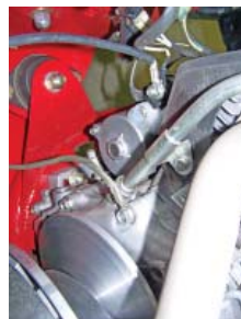
Solenoid positive cable connection.
